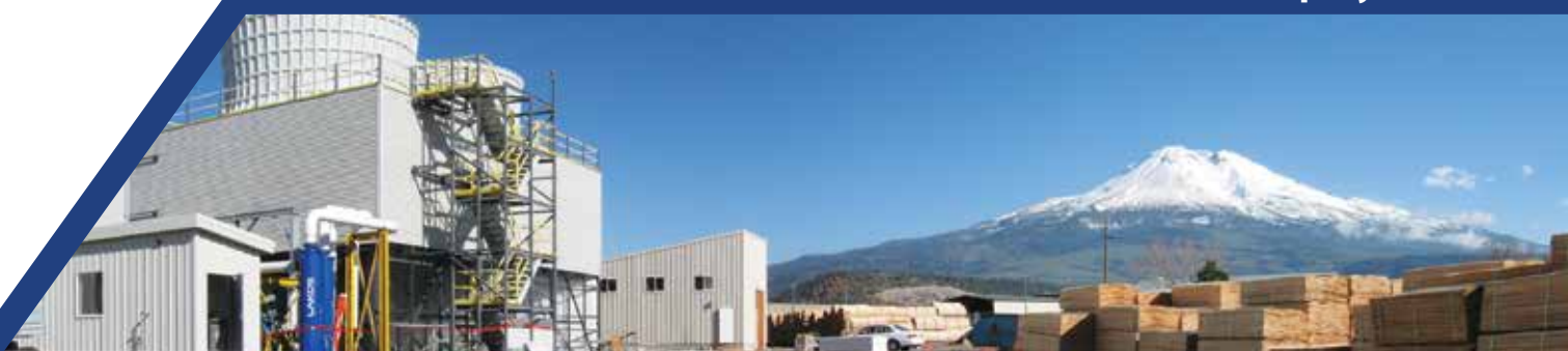
Prevent Solids Accumulation in Sumps and Basins
